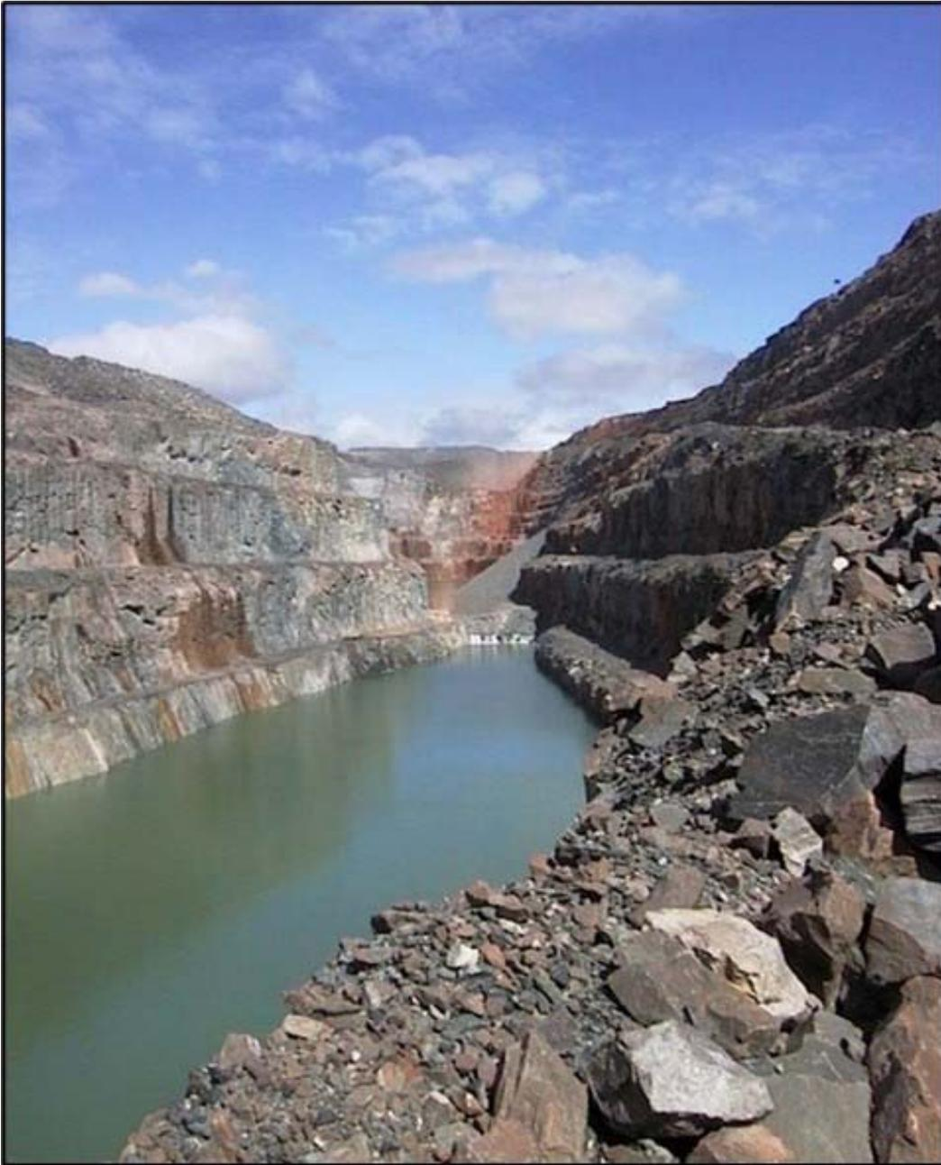
The Wenot Pit walls as shown in Figure 20.3 were stable. However, the upper section of the south wall was unstable, increasingly so, as the tailings pond water rose (Figure 20.4).
