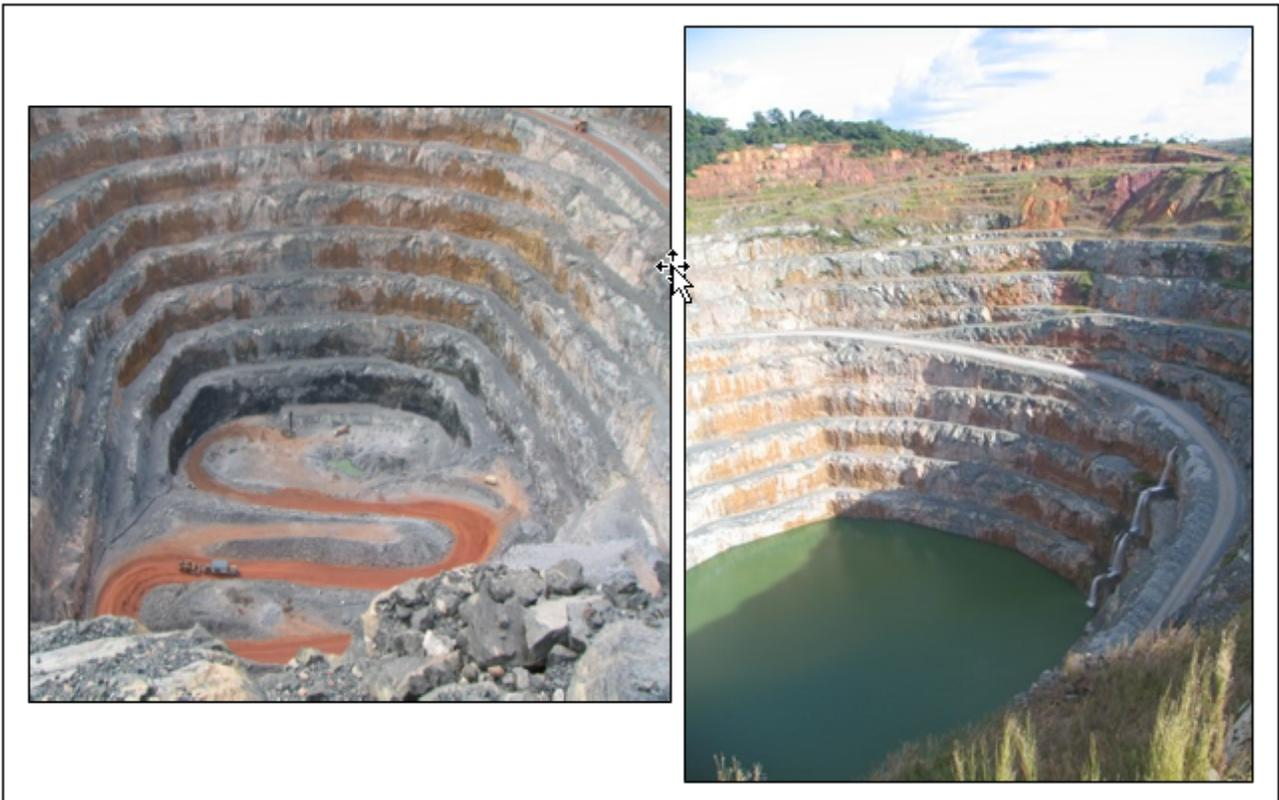
The Wenot Pit is shown in an east-to-west view in Figure 20.3, shortly after the initiation of tailings disposal into this pit in 2002. Over a period of 3 years, 21 Mt of tailings were deposited in this pit. Tailings discharge was from one point at the west end. As a result, the coarser tailings can be expected to have settled near the west end.
