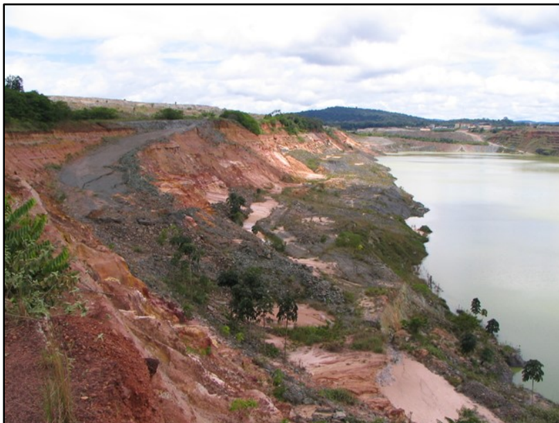
FIGURE 20.4 SLUMPING UPPER SECTION OF WENOT PIT SOUTH WALL, 2005
