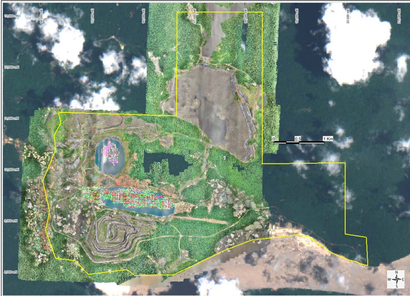
FIGURE 9.4 DRONE PHOTOGRAPH MOSAIC OF THE OMAI PROSPECTING LICENSE, LOCATION OF MINERALIZED AREAS
